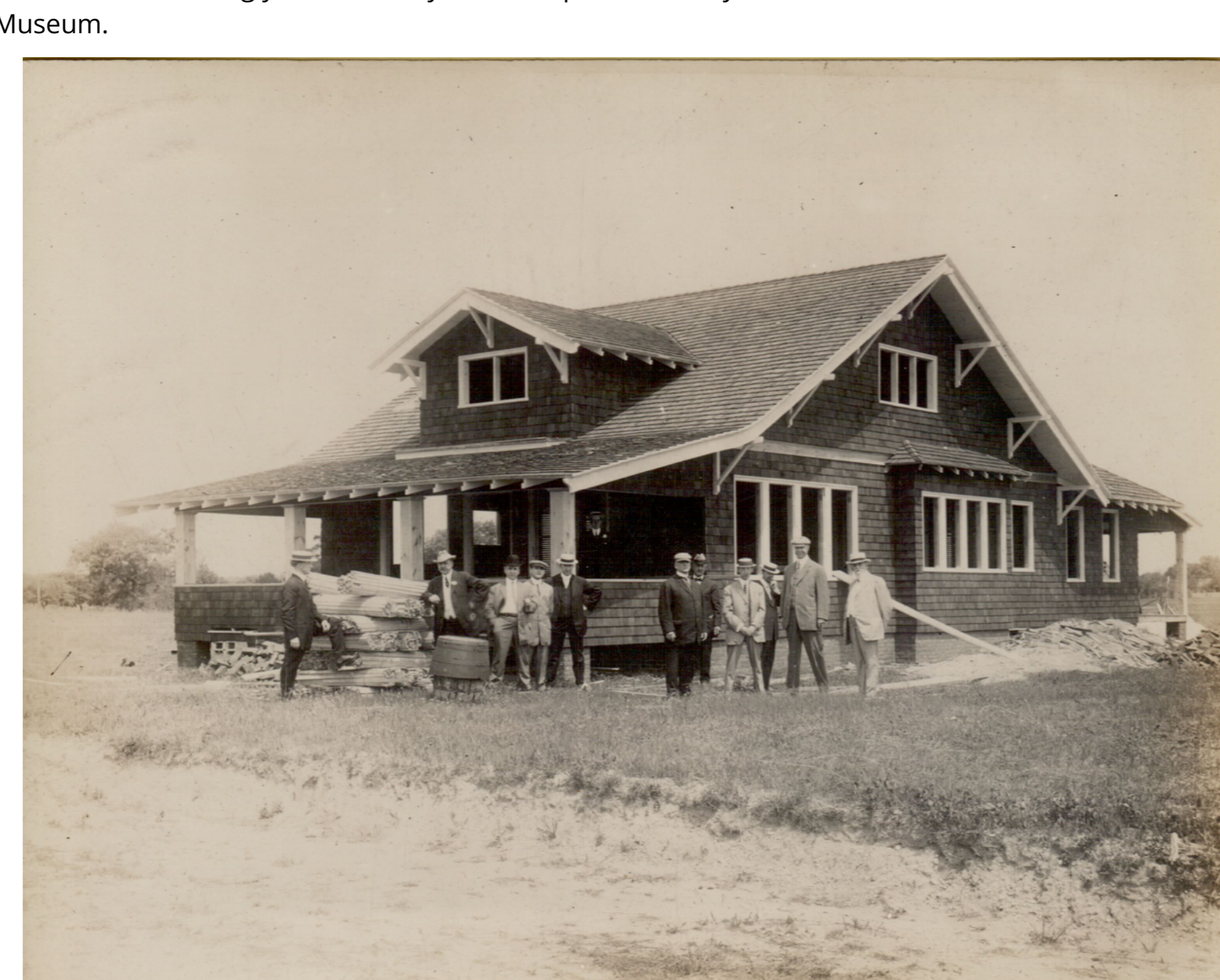
Here we see the Stone Harbor Country Club nearing completion and situated on the mainland at Cape May Court House. Please note the assemblage of men who are inspecting the progress of the ongoing construction of this soon to be officially opened club which would occur in mid-1911. In addition to a restaurant for fine dining and the ever-popular lawn tennis, there was a 45-acre 9-hole golf course also associated with this facility.
